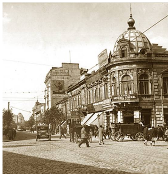
Figure 4. Construction in the 1930s
