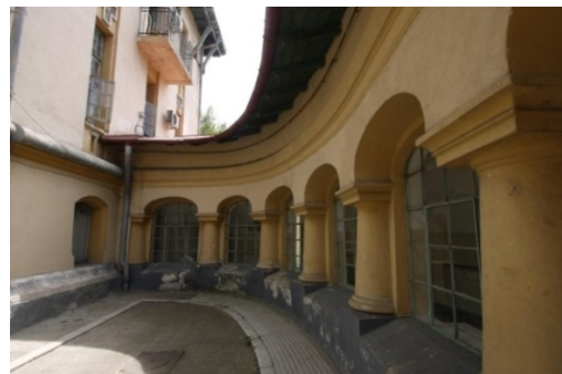
Figure 7. The curved walkway which connects the main wing to the kitchen's wing. Photo: 2012
