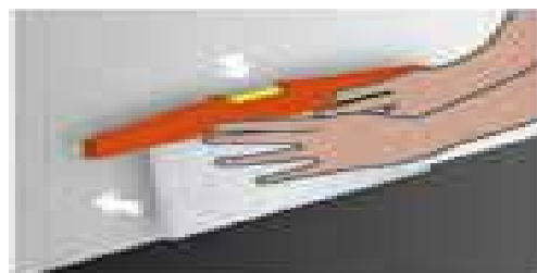
Positioning plate and check evenness
