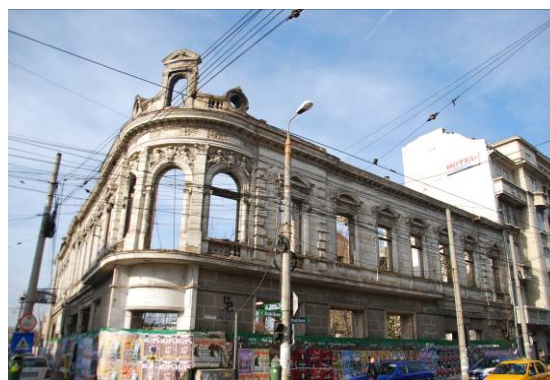
Figure 5. Construction in the 2010s
